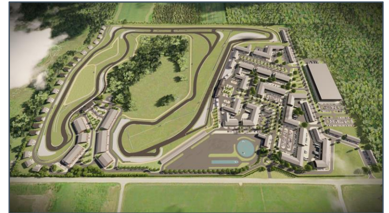
Oro-Station Innovation Automotive Park, Oro-Medonte (Simcoe County) Automotive engineering, field testing, education, and manufacturing businesses
