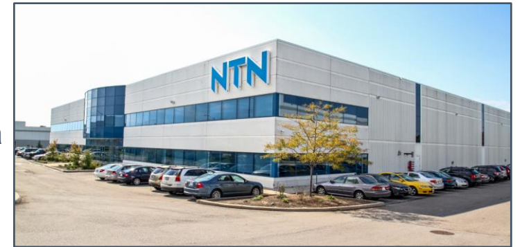
NTN Head Office and Warehouse, Mississauga
