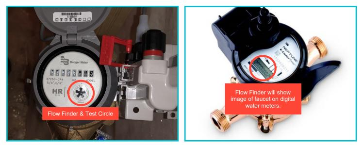
Above are two commonly used water meters in Middlesex Centre. If you suspect a leak, you'll want to check the dial called the "Flow Finder & Test Circle" (shown in red circle). These are very sensitive and are useful in determining whether or not a plumbing leak exists. If water is not running in your home under a regular situation and the black wheel is still spinning, you probably have a leak.
