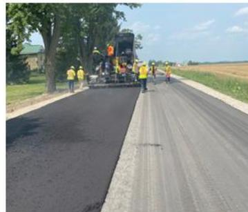
This project will resurface asphalt roads to maintain a Pavement Condition Index (PCI) of 70 or better as per the recommendations of the Asset Management Plan
